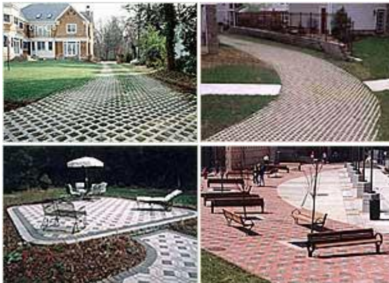
Figure 24.4 Examples of Porous Paver Surfaces
