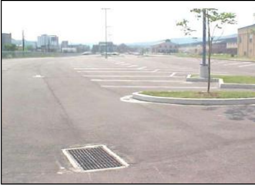
Grate Inlet in Parking Lot
