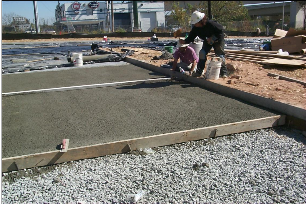
Figure 25.2 Porous Concrete System Installation
