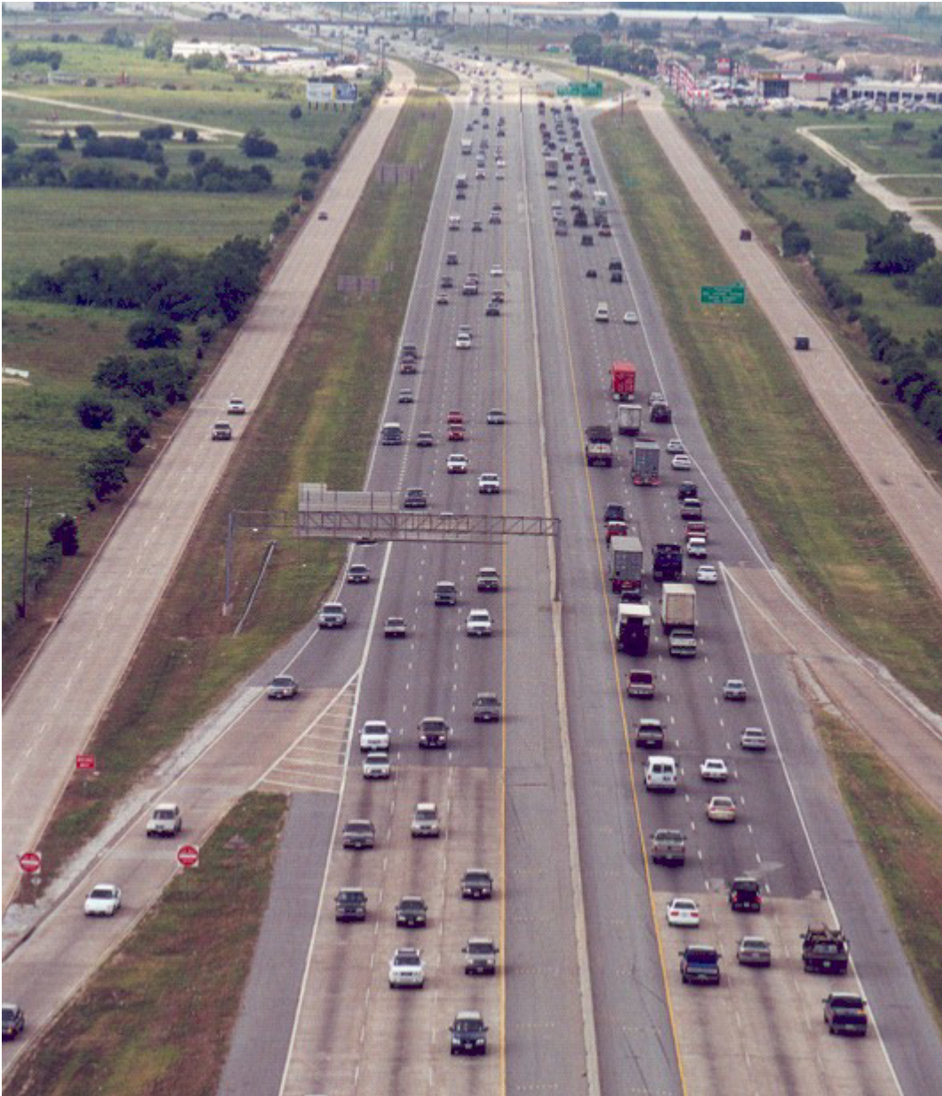
Figure 2-2. Freeway with Frontage Roads
